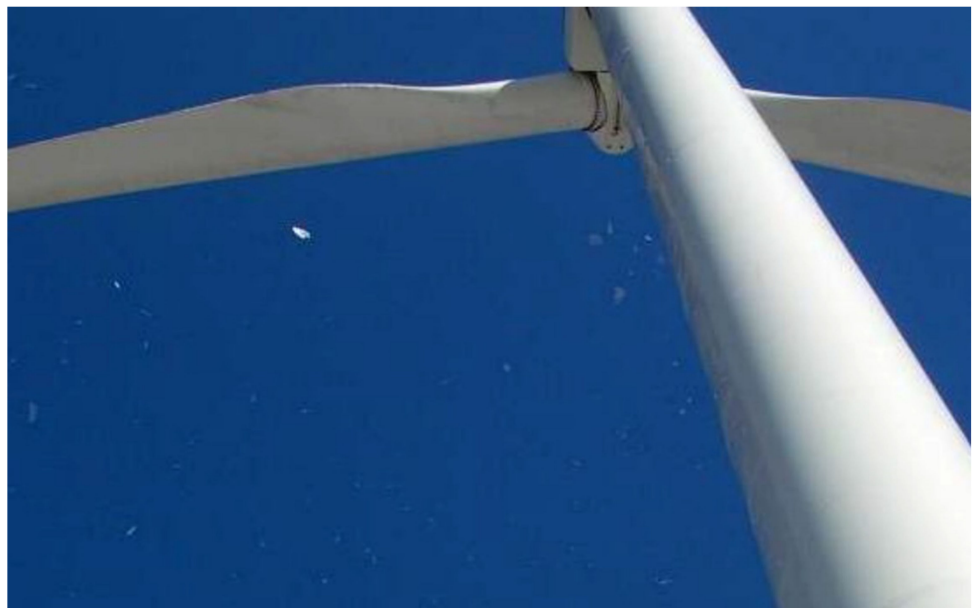
Figure 14. Ice falling or being thrown off a wind turbine poses a safety risk to turbine maintenance staff and, depending on turbine siting, the general public [69].
